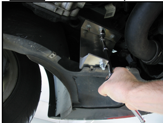
Picture G: Drivers side bracket fully installed.
