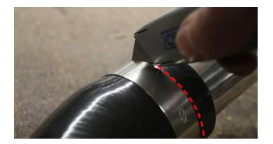
Cut around the silicone using the clamp as a guide to cut against. This will ensure you have a straight clean cut.
